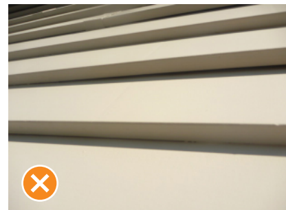
Figure 13 Gap of more than 2 mm between weatherboard laps on a light coloured painted wall.
