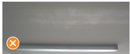
Figure 22 Sheen banding on a finished ceiling that is clearly visible from normal viewing position under non-critical lighting conditions. Source: Winstone Wallboards
