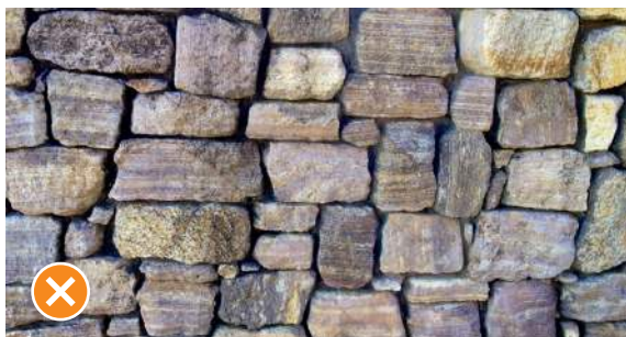
Figure 10 Stones are stacked on top of each other with continual running vertical joints and very little bonding. Source: NZSMA
