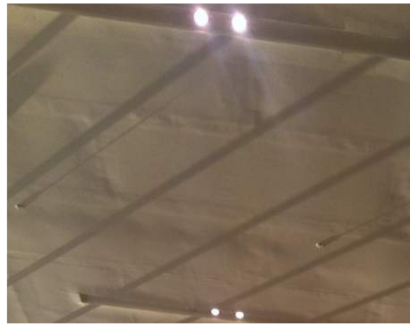
Figure 3 Critical lighting from low level sun on the same finished ceiling. Source: AWCIA NZ
