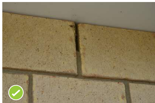
Figure 7 Ventilation openings are a requirement in a brick veneer.
