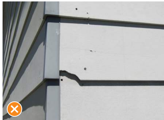
Figure 15 Damaged fibre cement weatherboard.
