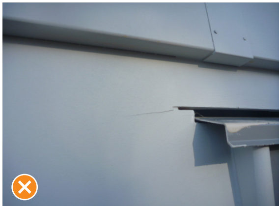
Figure 14 Crack in a fibre cement weatherboard.
