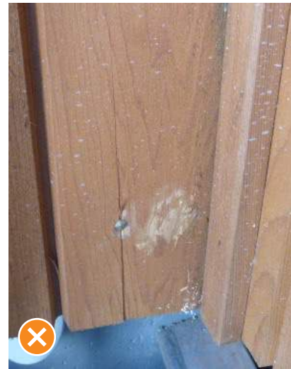
Figure 12 Split around fixing in a timber weatherboard.
