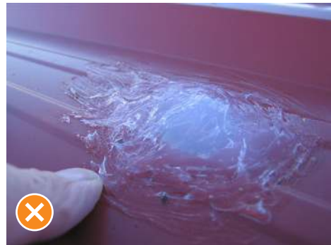
Figure 19 Sealant-filled fixing hole with untidy finish.
