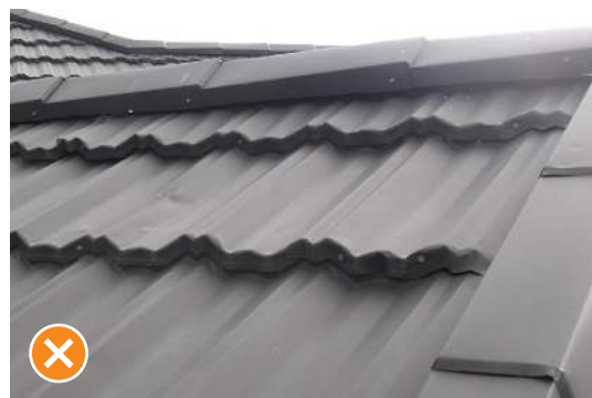
Figure 17 Dented metal tiles.
